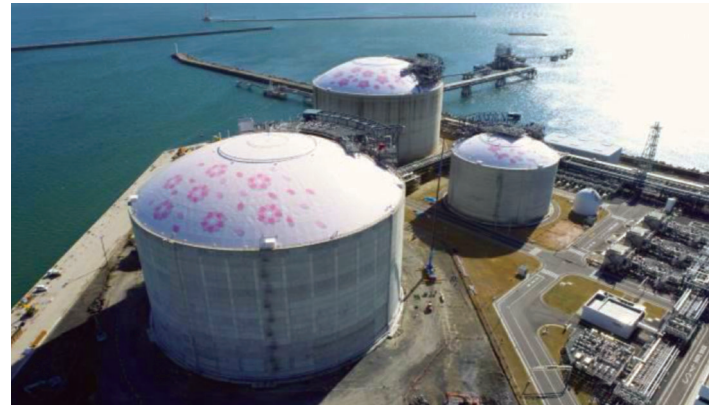
New Hitachi terminal tank is now in commercial operation
