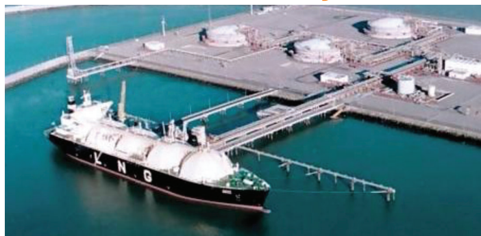
Das Island plant off Abu Dhabi has operated since 1977
