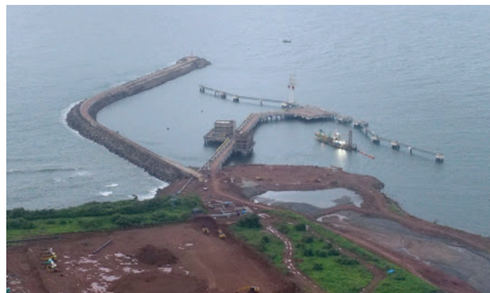
Port of Jaigarh in state of Maharashtra ready for FSRU
