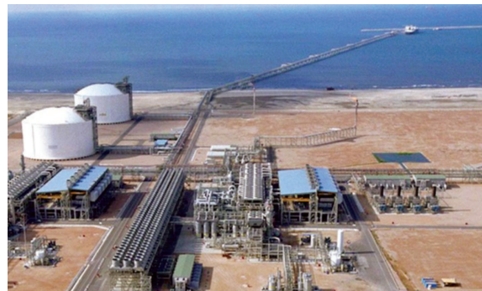
The plant near Alexandria has been idle since November 2012 because of domestic shortages now resolved
