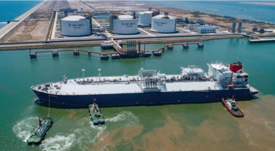
LNG carrier berthing at Tianjin regas terminal, operated by Sinopec
