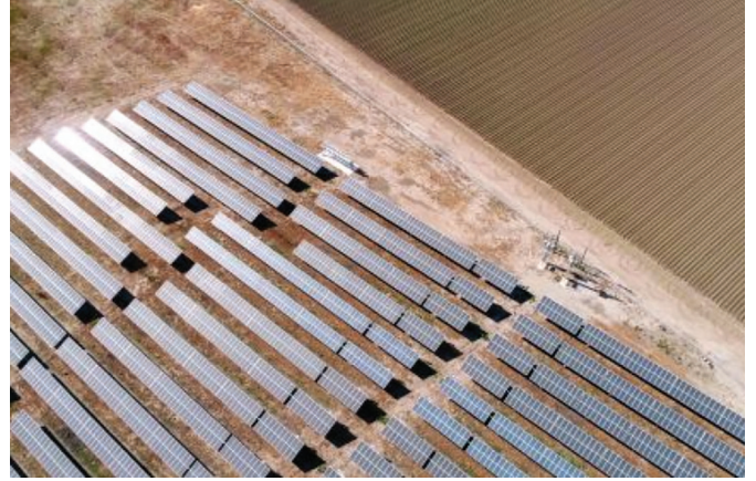
Large solar farm in Saudi Arabia
