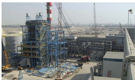
Construction of Jebel Ali L2 station
