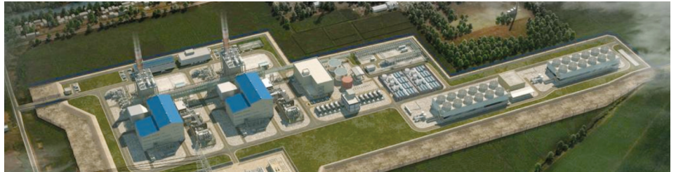
Render of Pertamina's Jawa-1 LNG-fuelled power plant (1,760 MW)
