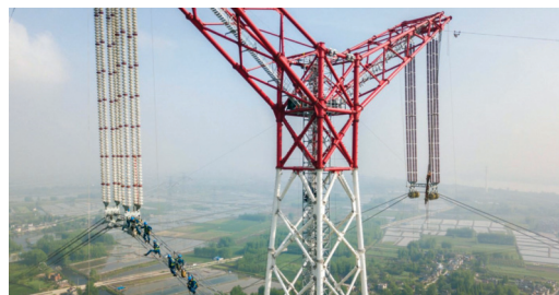
Ultra-high voltage power lines in China
