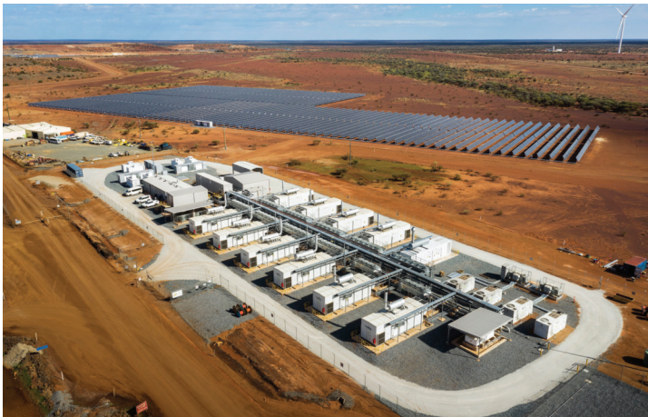
Bird's eye view of Gold Field's microgrid at the Agnew Mine
