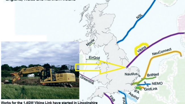
Works for the 1.4GW Viking Link have started in Lincolnshire
