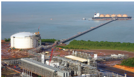
Cove Point LNG at the start of commissioning.
