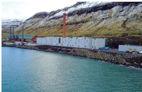
'Sund' power plant near Tórshavn, the Faroese capital
