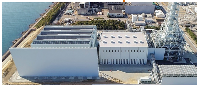
View of the new T-Point 2 with T-Point in the background at Takasago Works, Japan
