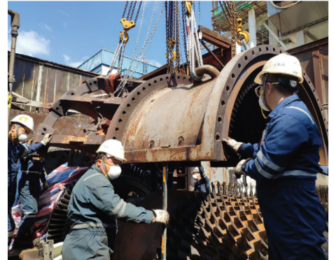
Works at the Baochang power plant in Shenzhen, China.
