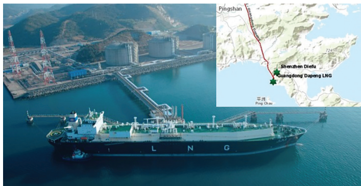
Shipments to CNOOC's Dapeng LNG terminal have surged
