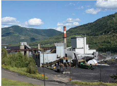
View of the Milner power plant near Grande Cache, Alberta.
