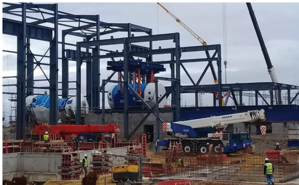
Installation of Ansaldo AE94.3A turbines at the Mornaguia site
