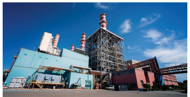
View of Torrevadalis Sud power plant
