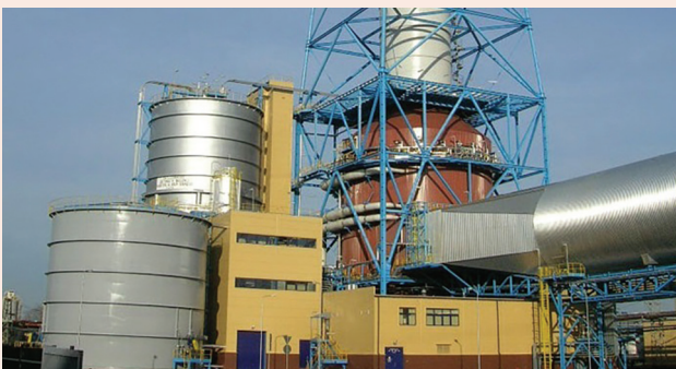
FGD system for Kozenice power plant in Poland
