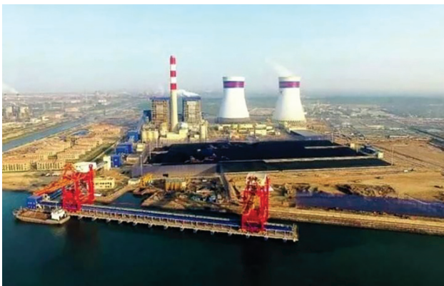
RLNG-fuelled Bin Qasim Unit 3 is being built next to two coal-fired units
