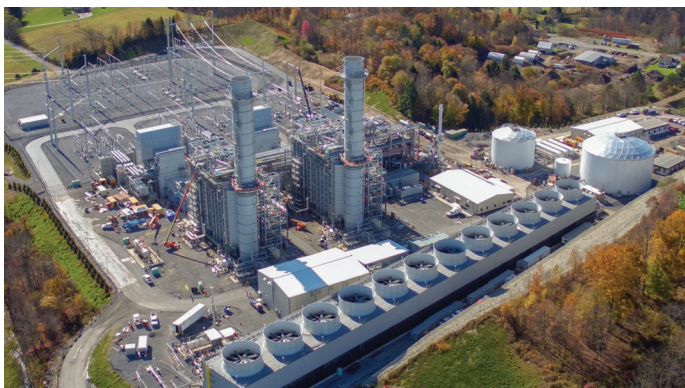
CPV's Fairview CCGT can now run on a 30:70 ethane and natural gas blend
