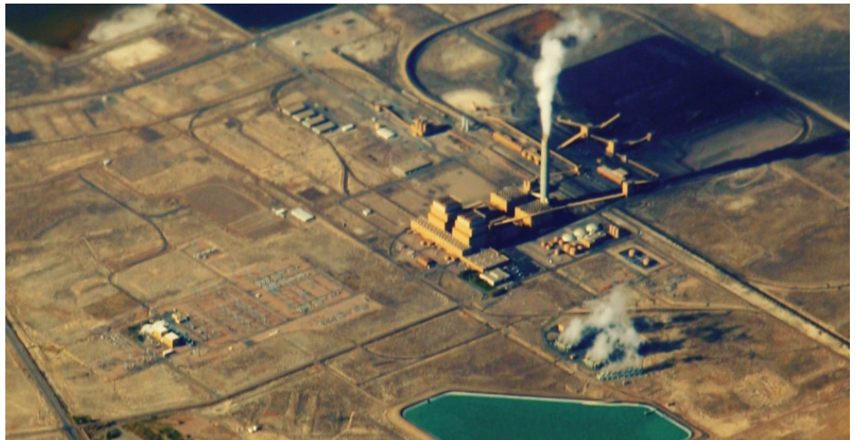
Bird's eye view of Intermountain PowerPlant in Utah
