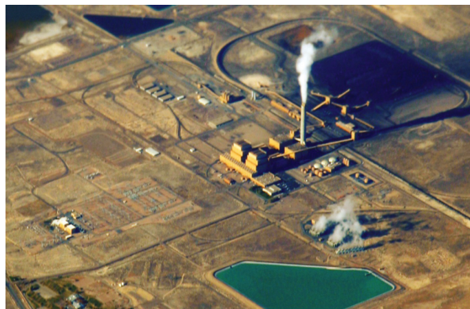
Bird's eye view of Intermountain Power Plant in Utah
