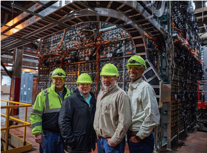
Greenidge team inside the peaking power unit
