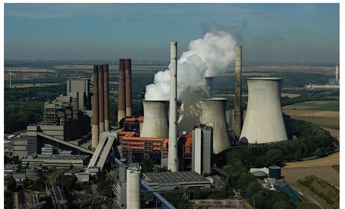
RWE's lignite power plant in Neurath
