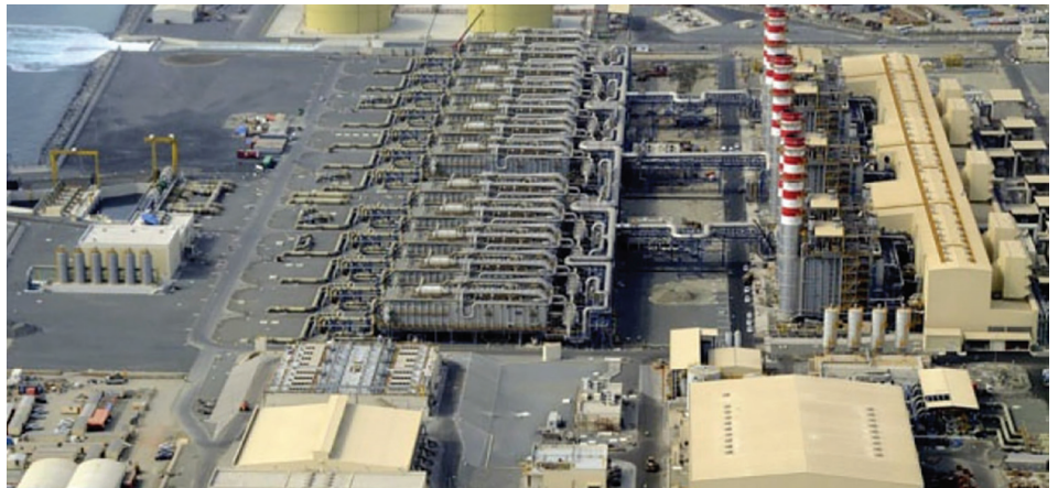
Fujairah F3 IPP will be built next to EWEC's F2 power and water plant
