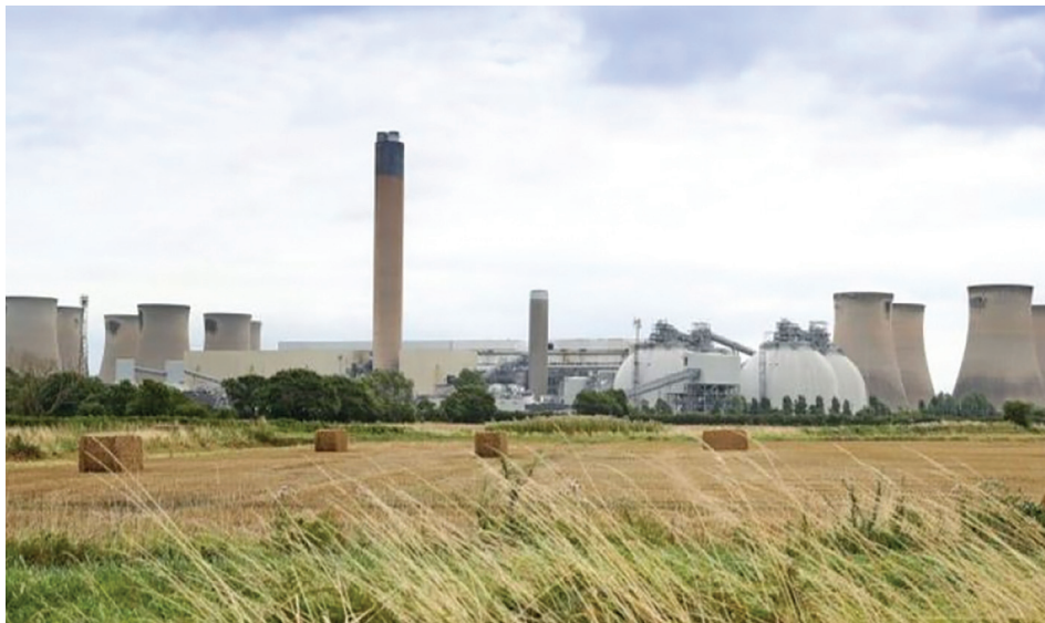
View of the 3.9GW Drax Power Station
