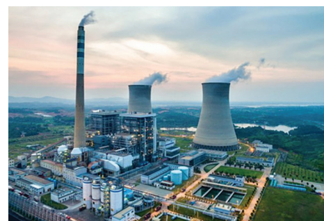
Şanlıurfa power plant
