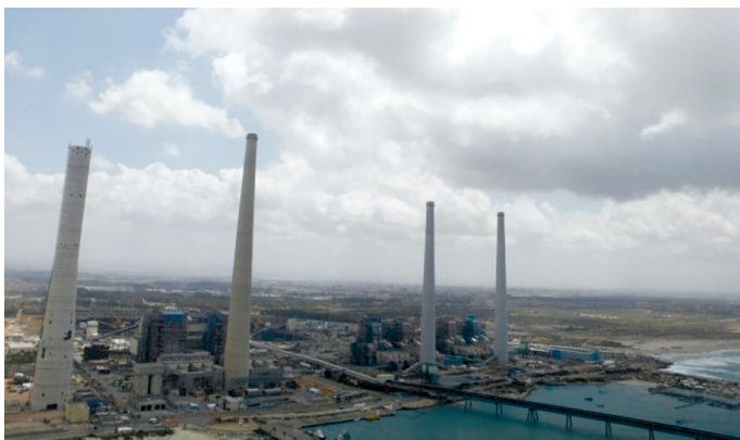
View of the Orot Rabin power station at Hadera, Israel.
