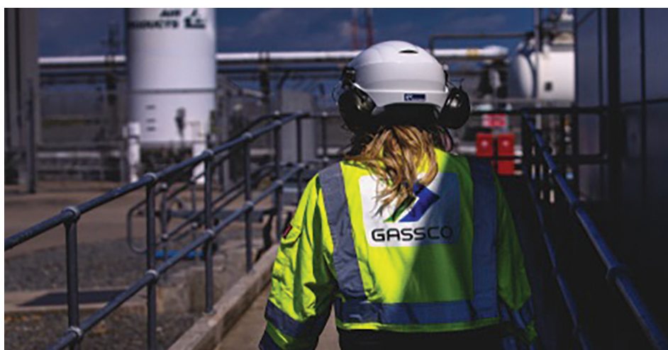
Langeled receiving terminal at Easington on the English east coast.
