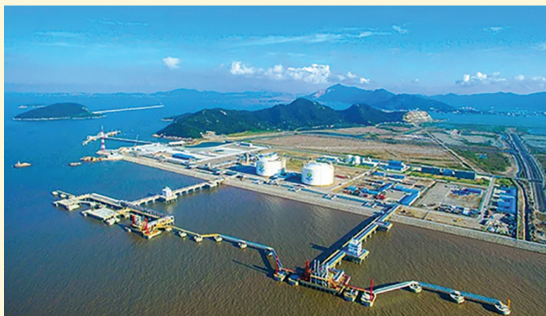
Zhoushan LNG regas terminal, operated by ENN
