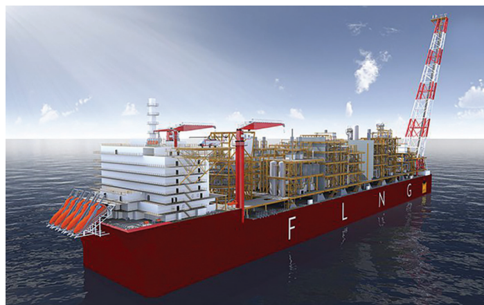
The hull of the giant FLNG was recently floated out of the building dock
