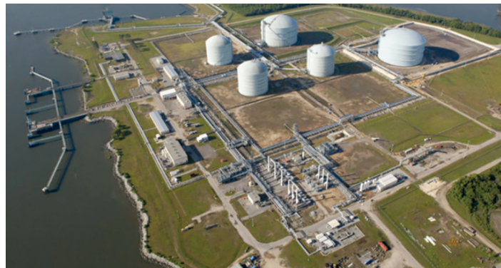
Commissioning starting on the eighth small-scale LNG liquefaction Train at the plant near Savannah
