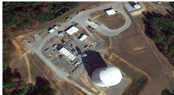
The small Pivotal LNG liquefaction plant in Alabama
