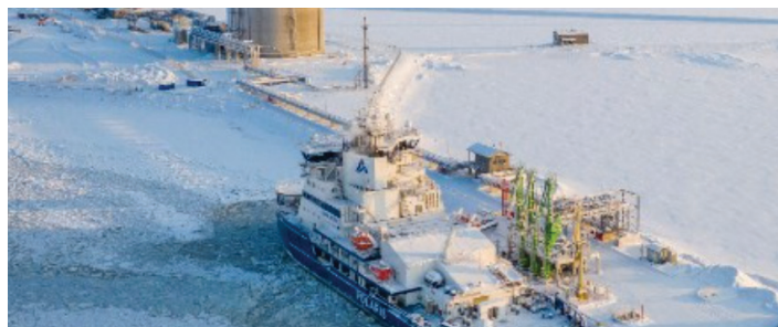
LNG regas terminal at Roytta harbour at Tornio in Finland
