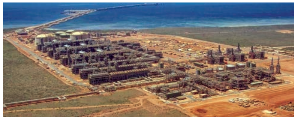
Australia's Gorgon LNG on Barrow Island has carbon dioxide injection system
