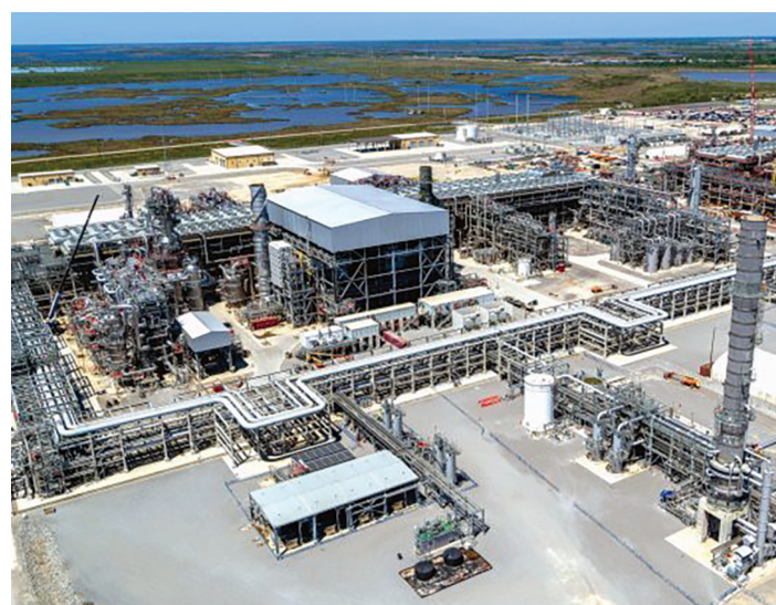
Cameron Train-2 during construction
