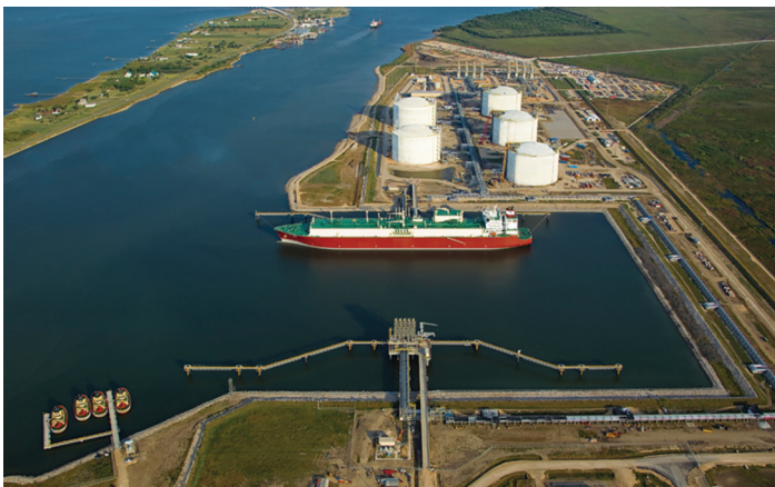
Construction of Golden Pass has commenced
