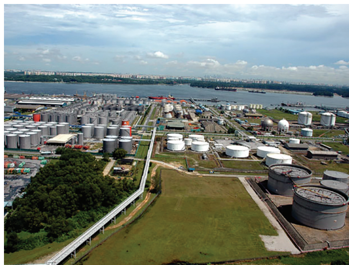
Johor is offering gassing up and cooling down services to the LNGC sector
