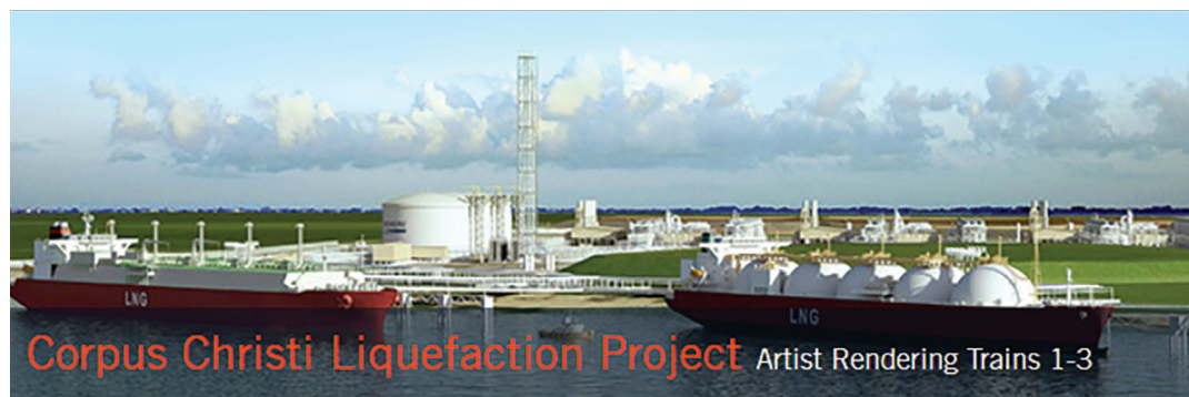
Cheniere's Corpus Christi Train 1 is 'substantially complete'
