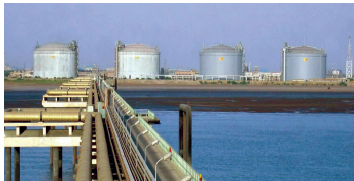
The Dahej import terminal located north of Mumbai
