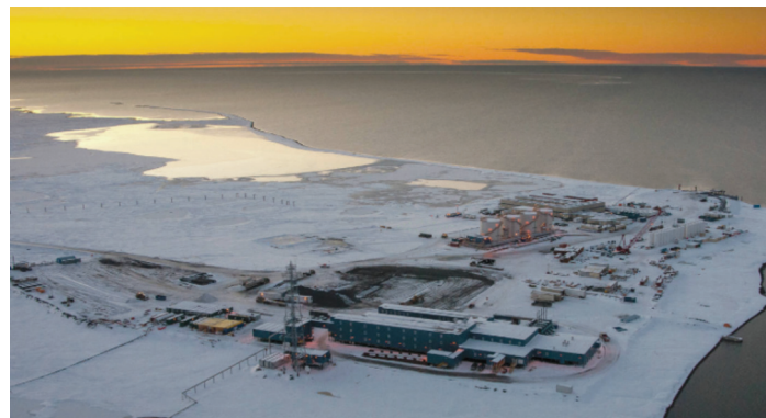
The Point Thomson energy facilities in Alaska's North Slope
