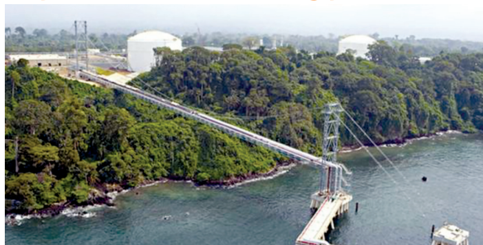
Liquefaction plant at Punta Europa on Bioko Island
