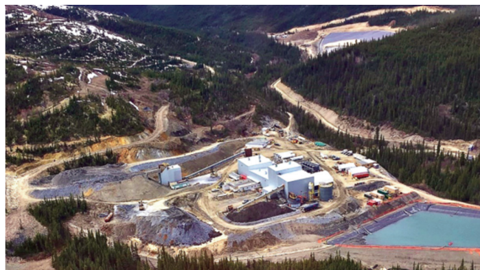
Cryopeak supplies LNG solutions to mines and remote areas
