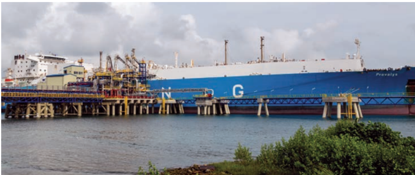
Operations at the AES-backed Costa Norte project in the Central American nation of Panama
