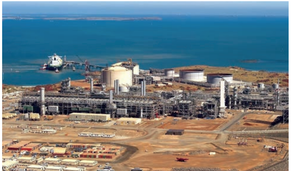
The Pluto plant will host the development of the Scarborough gas field now operated by Woodside. Four engineering contracts have been awarded
