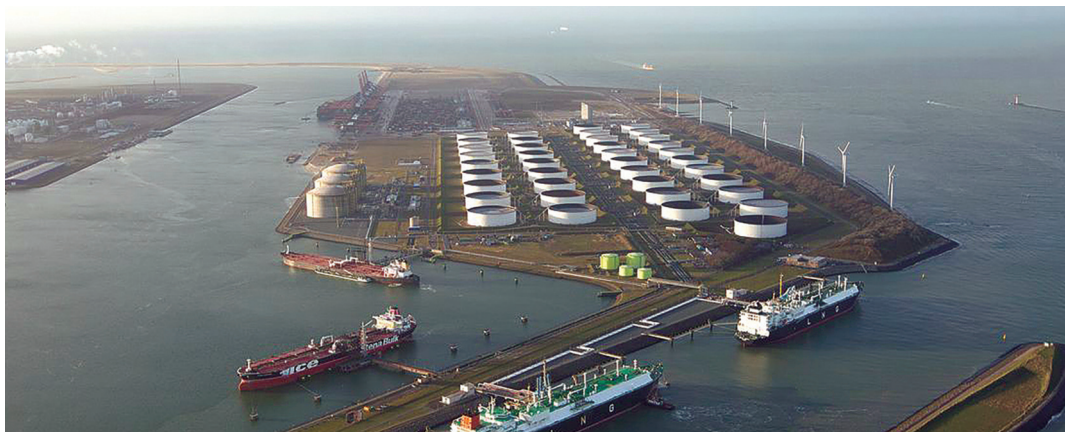
Gate terminal, Rotterdam
