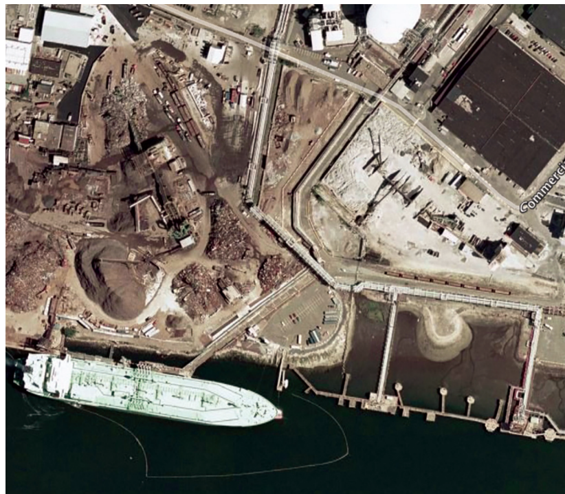
Bird's eye view of Everett LNG terminal
