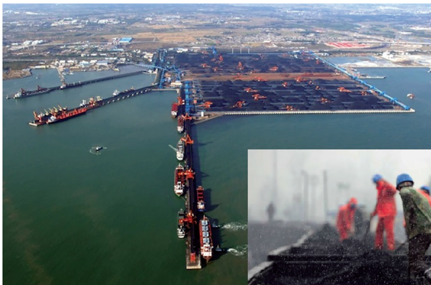
Coal terminal at Qinhuangdao maritime port
