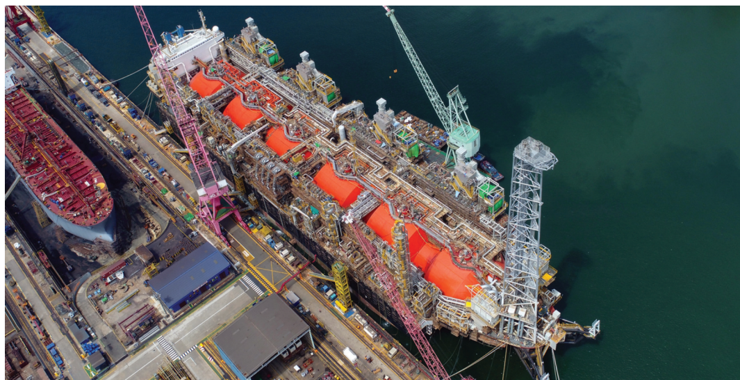
'Hilli Episeyo' seen undergoing conversion to an FLNG at Keppel
