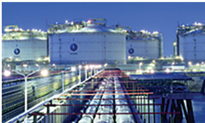
KOGAS is looking to build another receiving terminal
