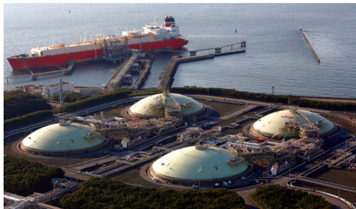
A Jera cargo arrives at the Futtsu import facility near Tokyo
