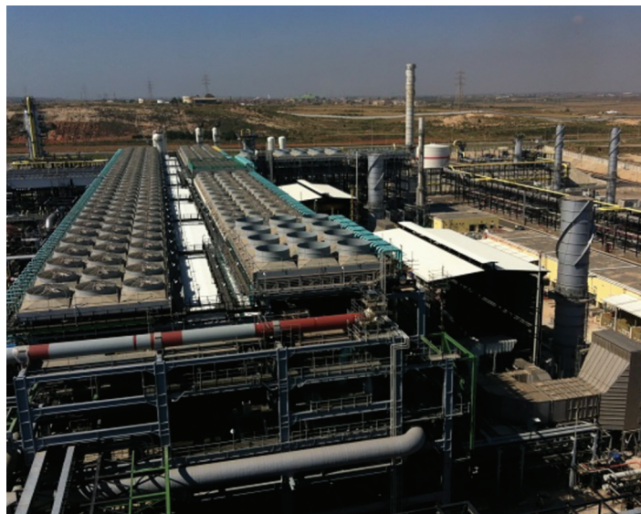
Project centres on Sonatrach LNG Trains at port of Arzew
