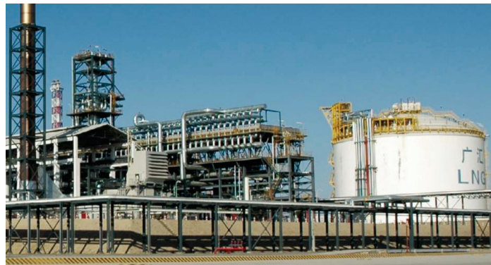
Plant built by German firm at Xin Jiang in northwest China
