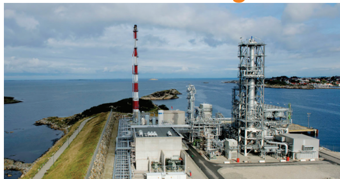
Skangas assets include the small-scale Risvika plant
