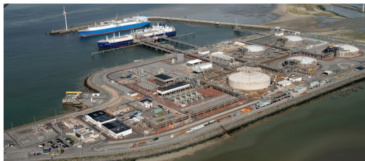
Zeebrugge transfer between Ice-class carrier and convention vessel
