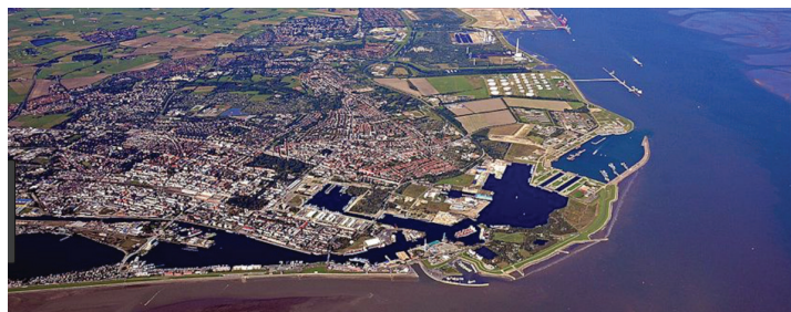
North Sea port has large area for LNG terminal plans
