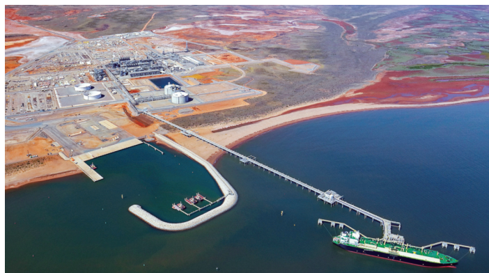
Wheatstone plant in Pilbara area of Western Australia
